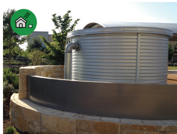
RAINWATER CAPTURE, STORAGE, FILTRATION: Cistern, pond, or underground tank designed to collect rainwater. Filtration system to remove contaminants, so the water can be reused on-site during boil water notices.
